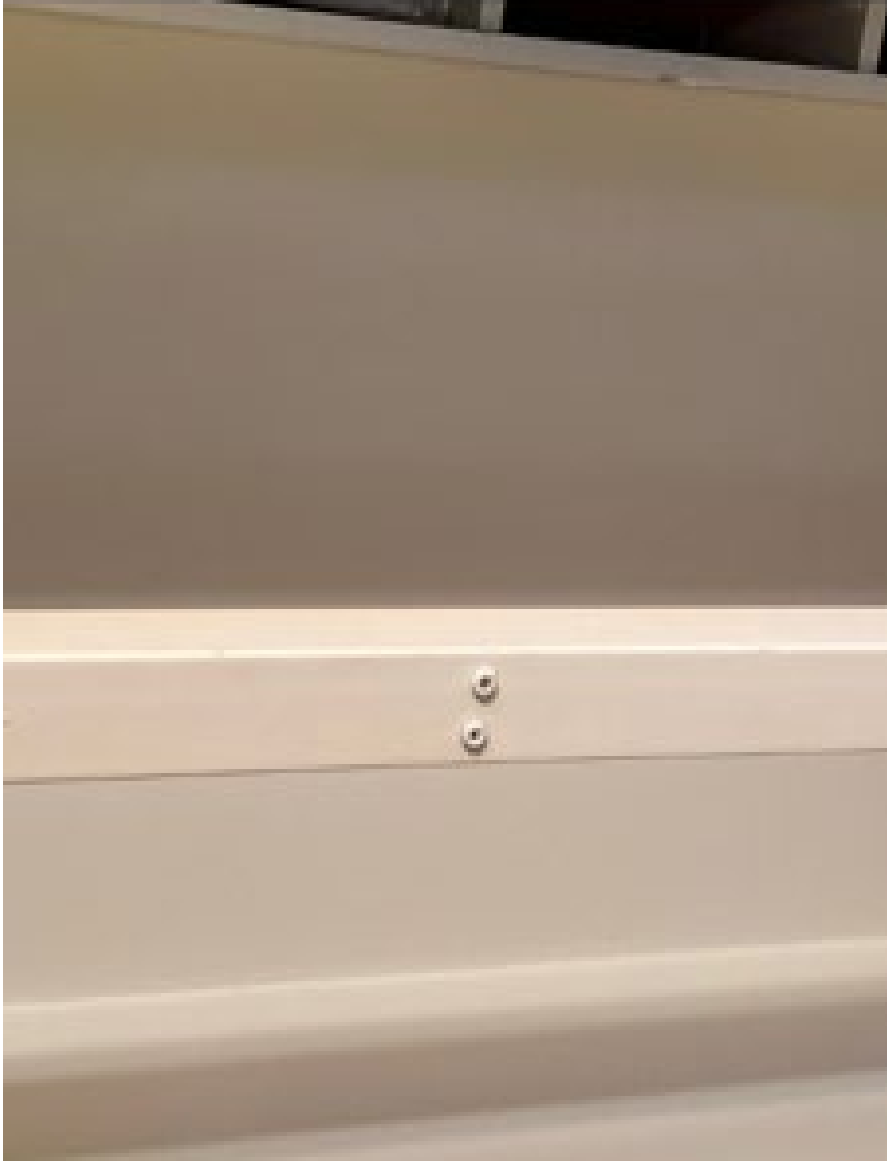
Final product of restoration activities
